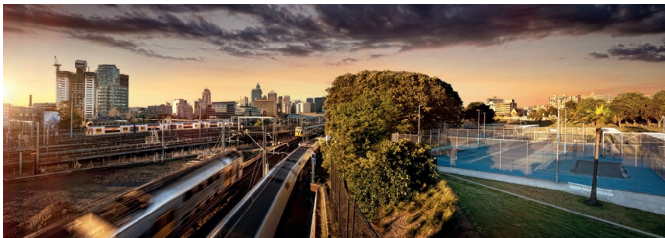
City infrastructure: rail lines, shade trees and tennis courts, Prince Alfred Park, Surry Hills. Photo: Joseph Nalevansky.
